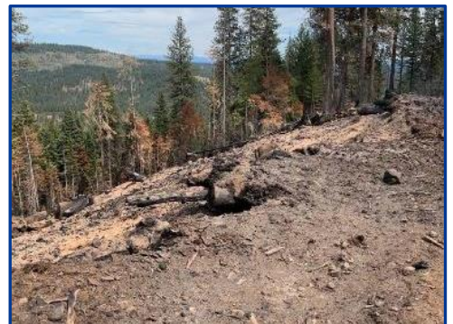
Photos taken of the roadbed and other ash pits showing how the logging slash burned out under the road in a cornice-like drop off.
